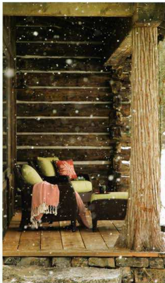
Opposite: Lone Chief features salvaged and reclaimed wood, much from local barns, supplied by Wild Wood Eccentrics. Interior trim and doors are also of reclaimed wood, mostly locally plentiful fir and larch. Above: Outside bark-on cedar posts frame the hewn logs, stone and cedar materials.
